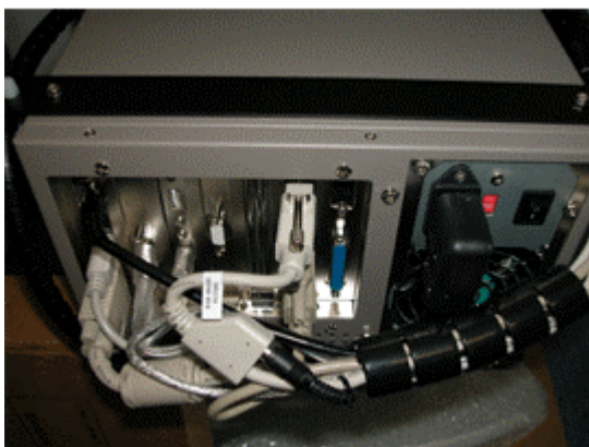
Figure 3: Equipment connections below the PC.
